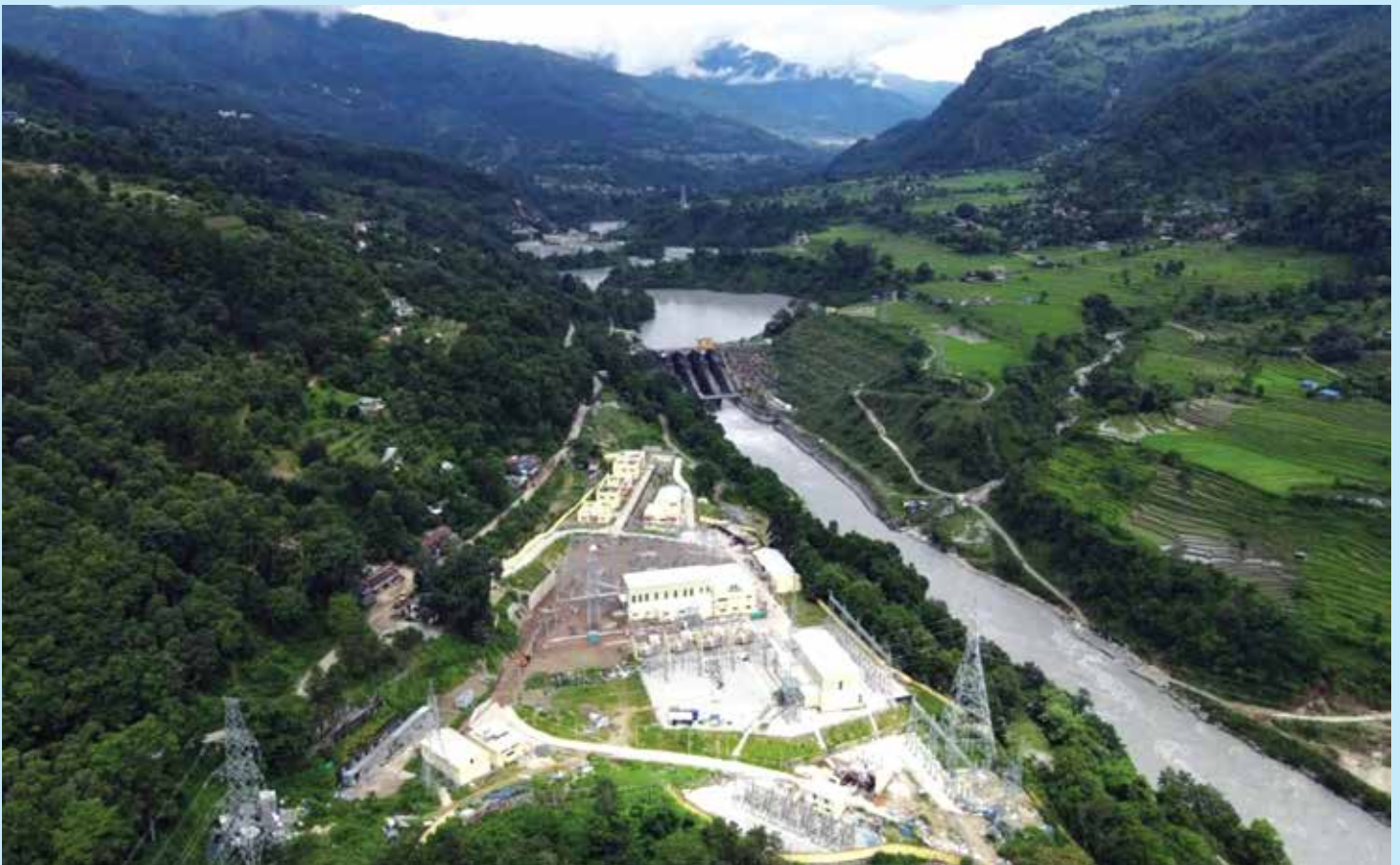
Recently Completed Udipur Substation in Lamjung District
