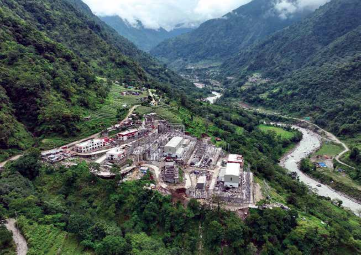
Under Construction Khudi Substation in Lamjung District
